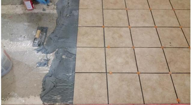
Figure 3 – Mortar and tile partially installed over concrete slab
